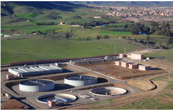
Caption: Completion of equipment installation ahead of commissioning
