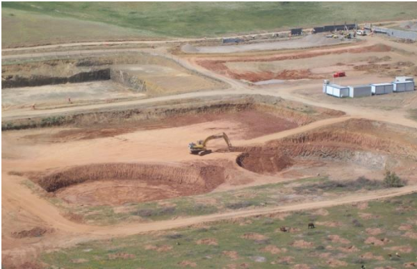
Caption: Initial construction works commencing
