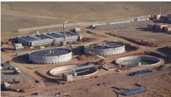
Caption: Equipment installation
