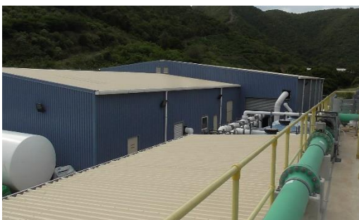
Caption: Reverse osmosis hall, chemical building and carbon dioxide tank
