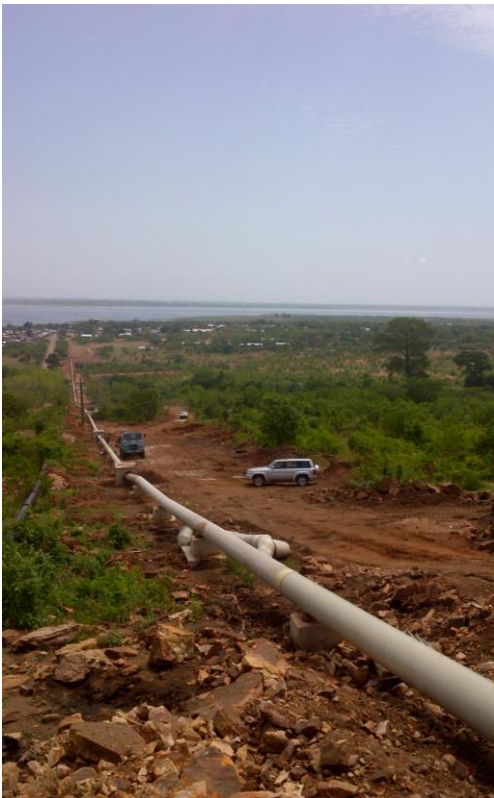
Caption: Installation of pipe support plinths above ground
