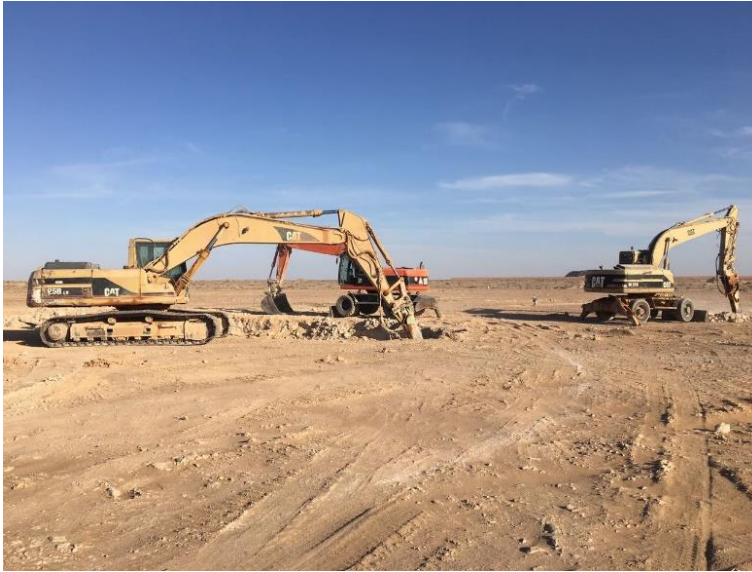
Caption: Laayoune Wastewater Treatment Plant Earthworks
