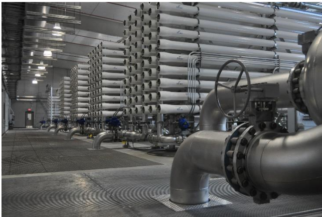
Caption: Reverse osmosis hall
