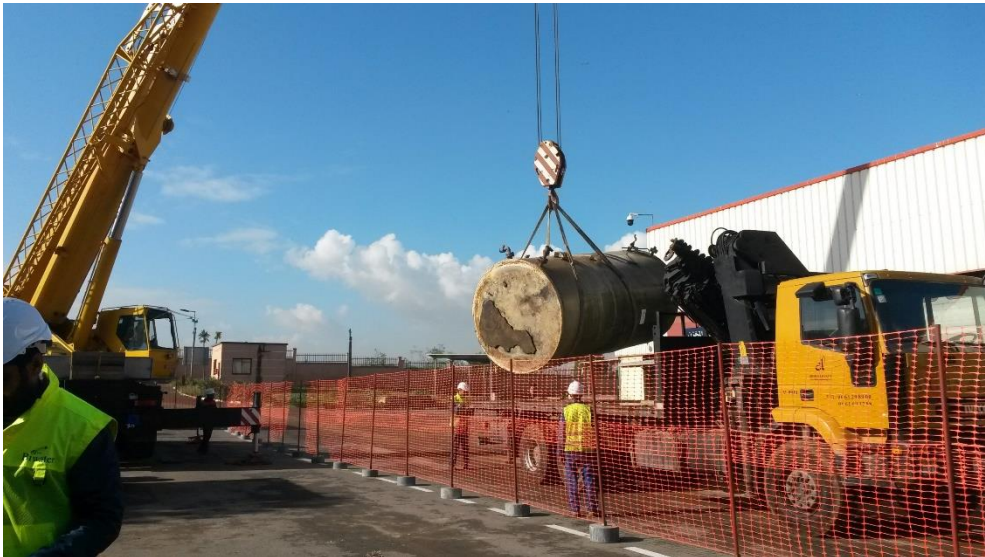
Caption: Removal of chemical storage tank for return to client's consolidation yard
