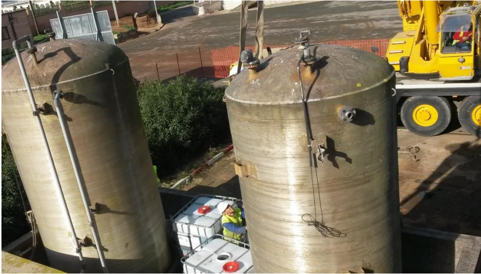
Caption: Biwater team removing chemical storage tank
