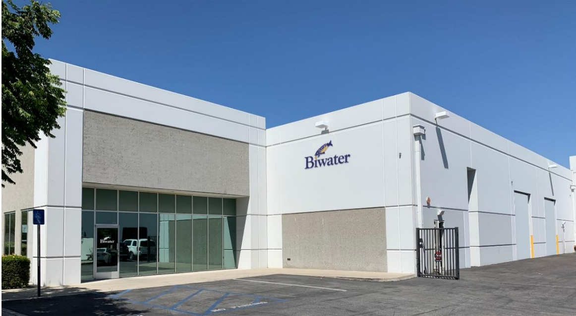
Caption: Biwater Inc's. new facility in Rancho Cucamonga, California
