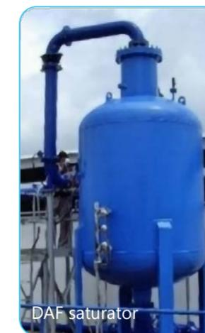
Water enters the DAF zone via a drop box that directs flow to a riser channel, where it contacts with an air saturated recycle stream. When released, at reduced pressure, this air saturated stream results in the formation of microbubbles that “sweep” up fine neutrally buoyant and colloidal material to the surface of the flotation zone for subsequent hydraulic descumming.
