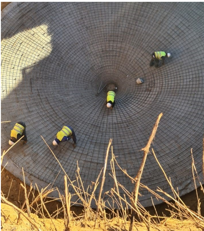
Caption: Moulay Bouselham Wastewater Treatment Plant construction in progress
