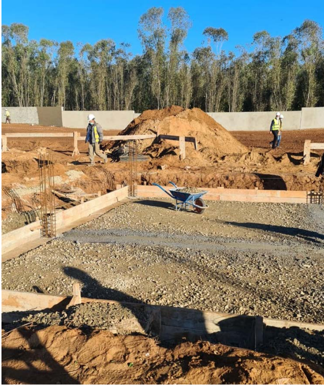
Caption: Moulay Bouselham Wastewater Treatment Plant construction in progress
