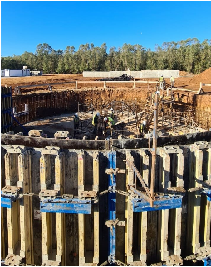
Caption: Moulay Bouselham Wastewater Treatment Plant construction in progress
