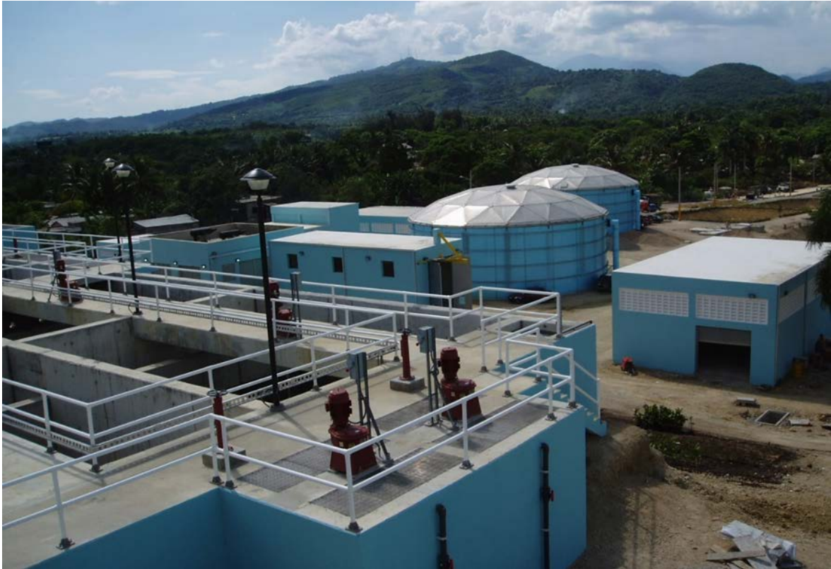
San Cristobal Water Treatment Plant under construction in the Dominican Republic
